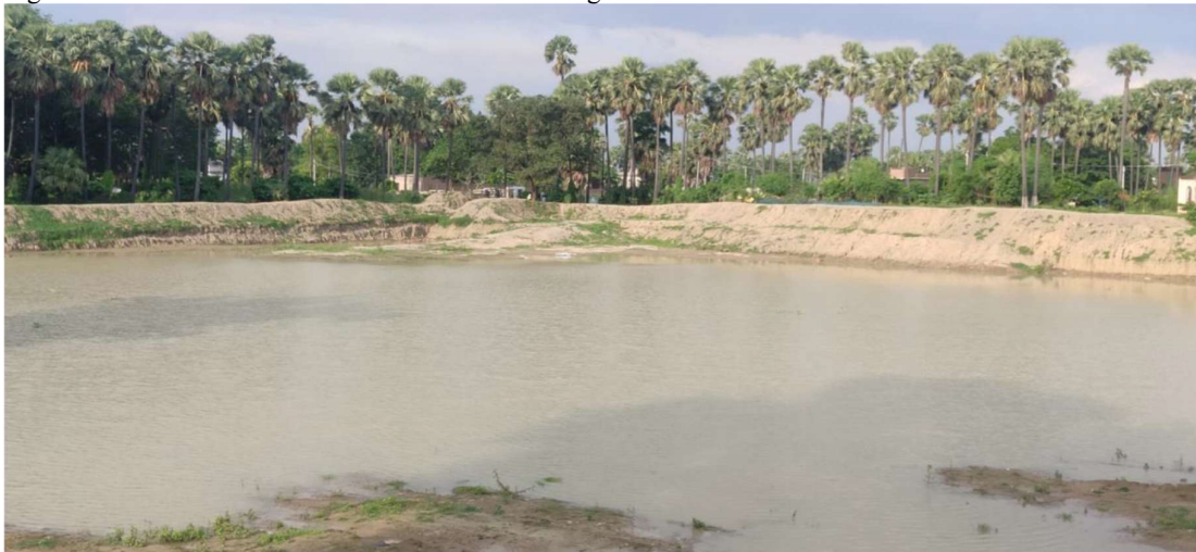
Figure 5. Rainwater Reservoir to Collect and Discharge into Groundwater.
